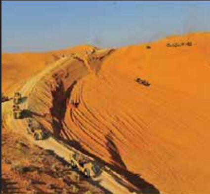
EARTH AND ENABLING WORKS
